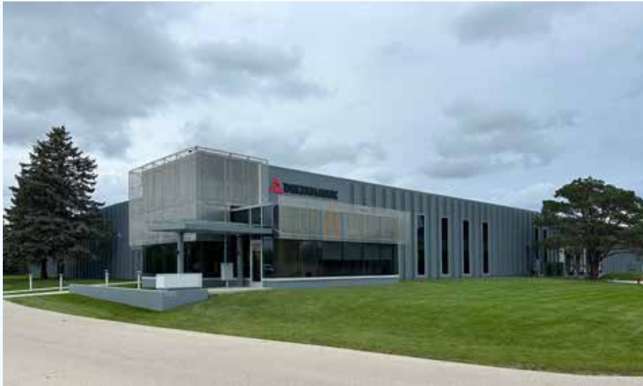
DeltaHawk's office and engine assembly facility at Racine International Airport.
